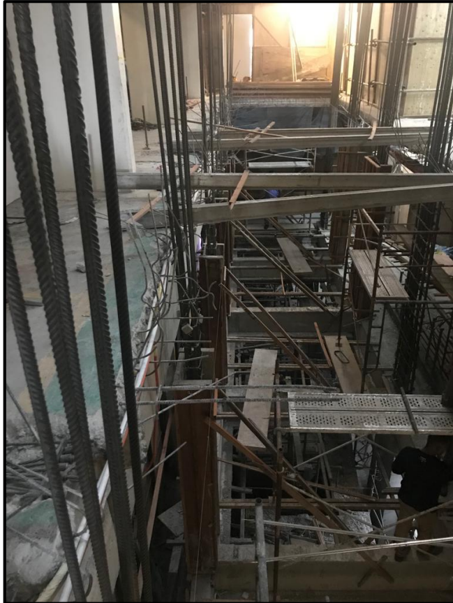
Casting of lift shaft in progress
