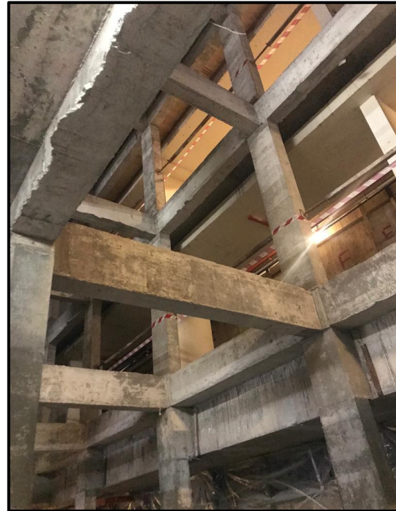
Casting of lift shaft (beams, columns, and slabs) in progress
