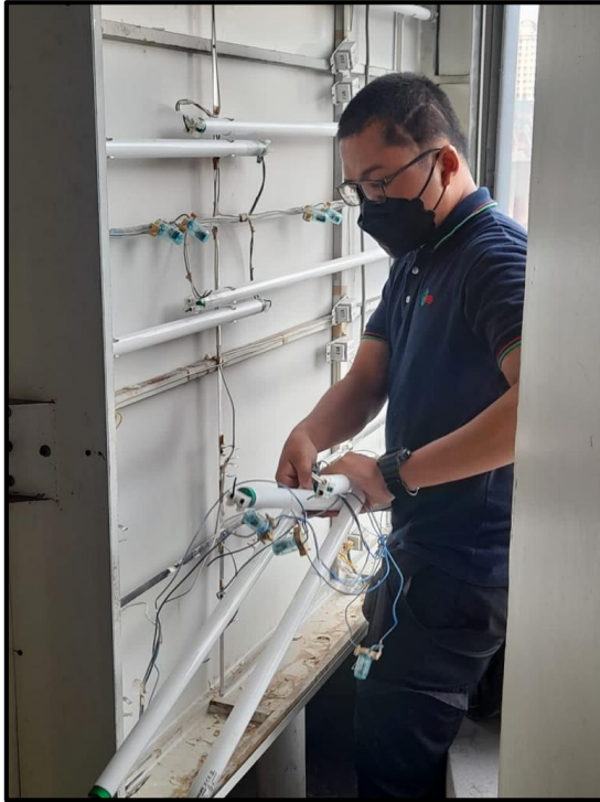
Previous Arrangement 12 Fluorescent Lights Total 324W per panel
