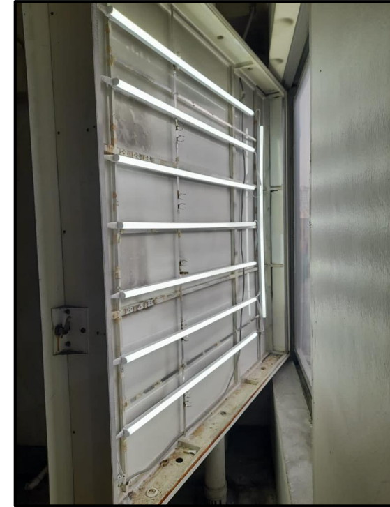
New Arrangement 8 LED Lights Total 104W per panel
