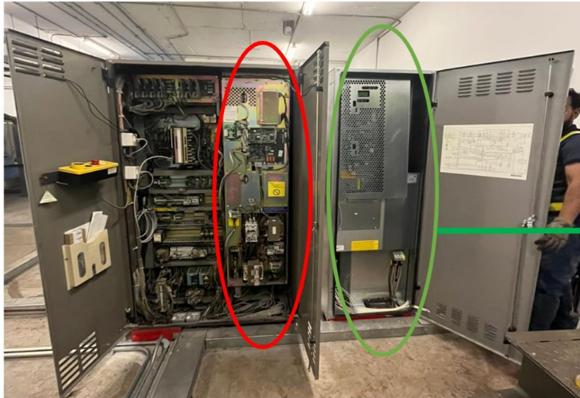
OLD INVERTER (in red circle) , NEW INVERTER (in green circle)
